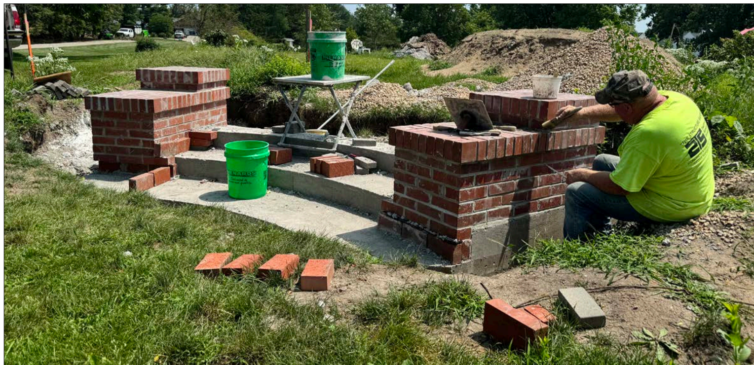
Technical Specialty Systems working on the brick steps and foundation as part of the Night Garden Restoration.
