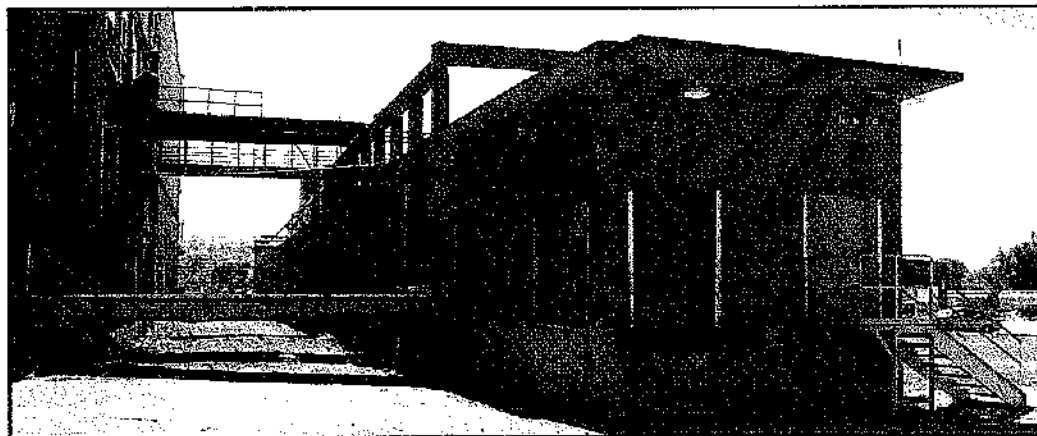
#60 Central Loading Dock, looking southwest (top) and looking southeast (middle); #69 Refrigerated Track Dock, looking east (bottom)
