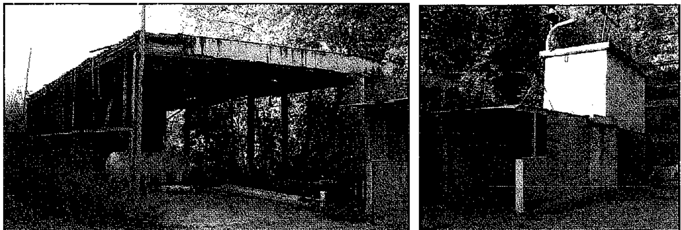
#71A Flotation Basin, looking southwest from service drive
