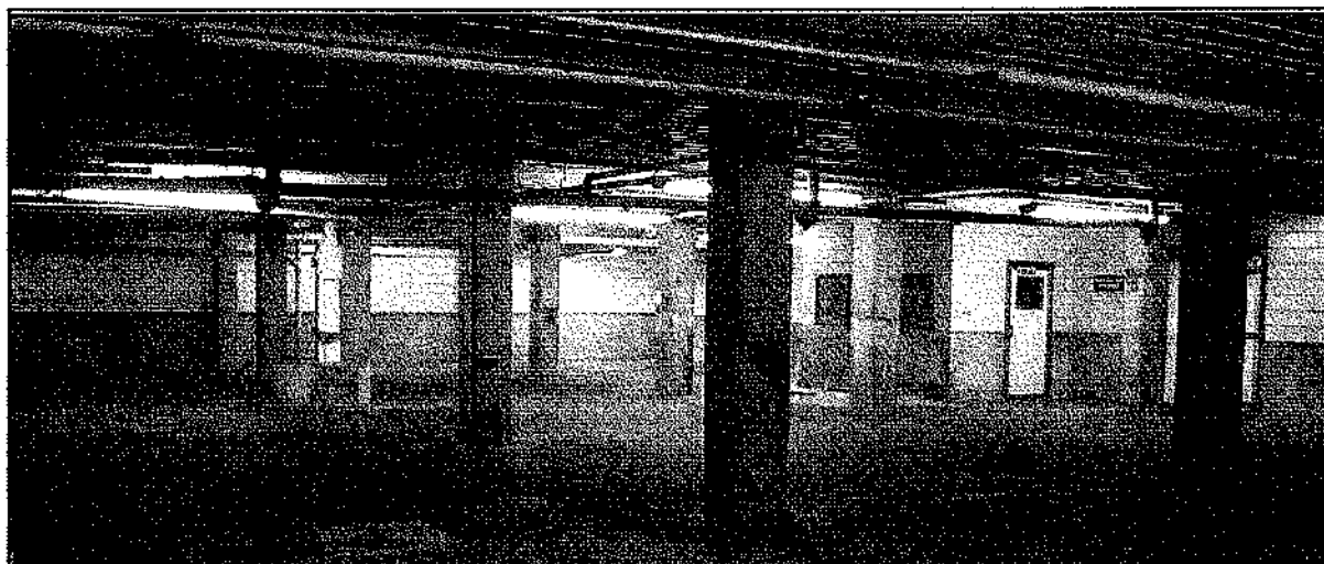
Building #23, first floor, looking southeast
