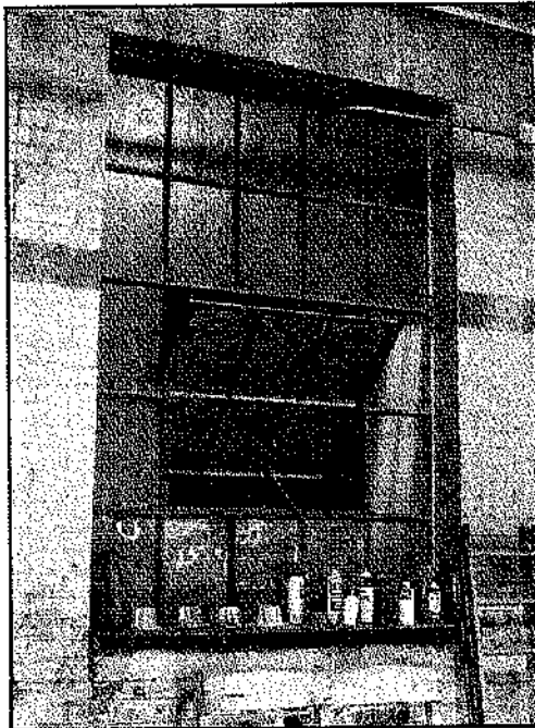
#9 Main Garage, original window, north wall
